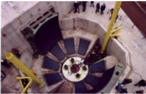
Building up new barrier
